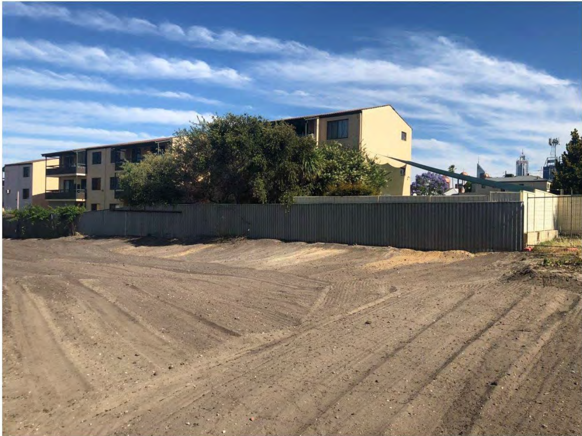
3 Storey walk up flats in the south.
