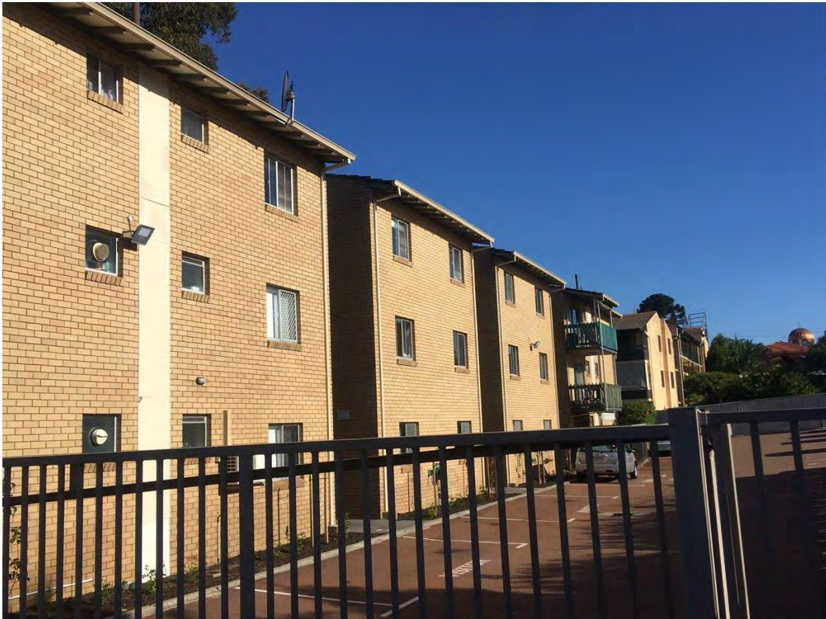
3 Storey Flats showing elevation viewed from East end of subject site
