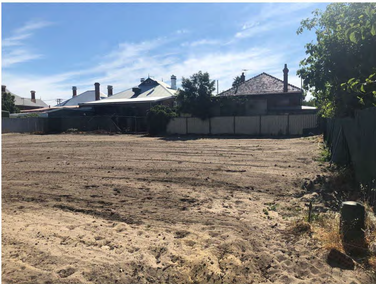
View into site where lane is to be extended and townhouses to be built
