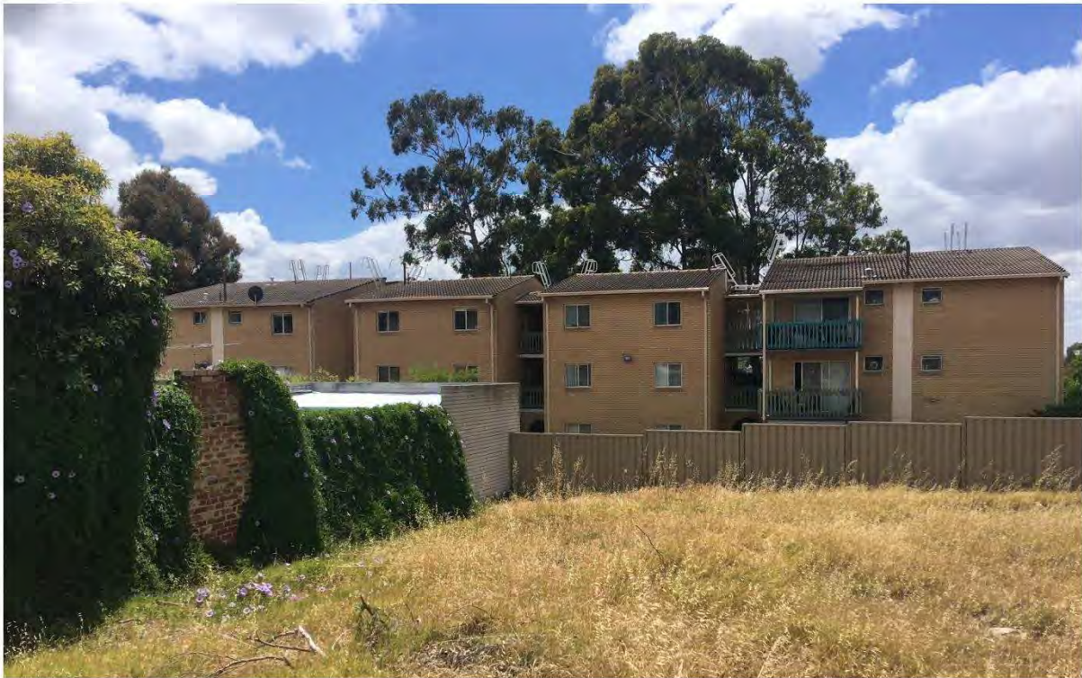
View east towards three storey walk up flats
