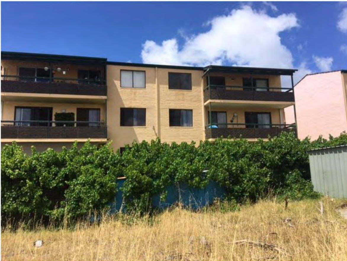
View from site to the south elevated 3 storey walk up flats with overlooking encroachment.
