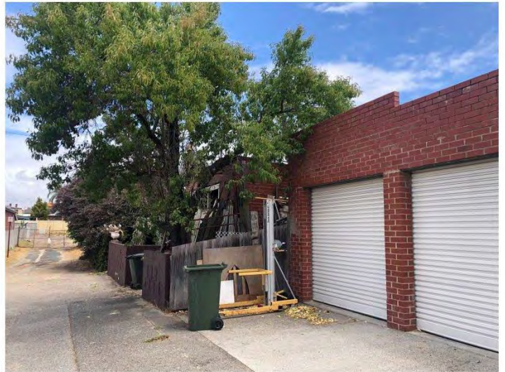
Sheridan Lane –approach to Lane extension
